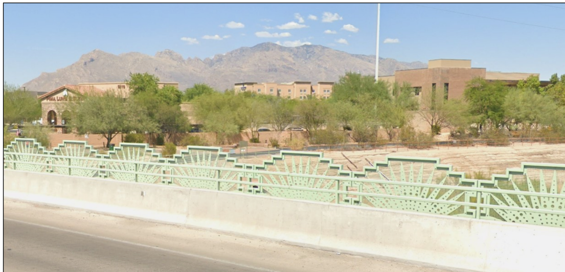
Figure 11. Decorative metal barrier on La Cholla Boulevard Bridge
